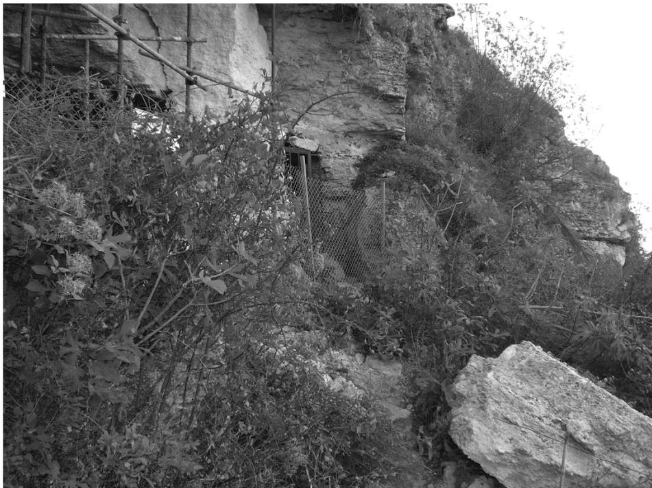
Figure 4 Breakdown at the entrance of St. St. Constantin and Elena Rock Church after the Kamen Bryag earthquake in 2009 (photo K. Kostov)
